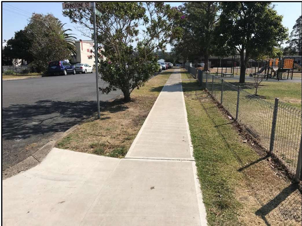
Photo 2 – View north along Johnstone Street showing footpath adjacent to school to connect to Waugh Street
